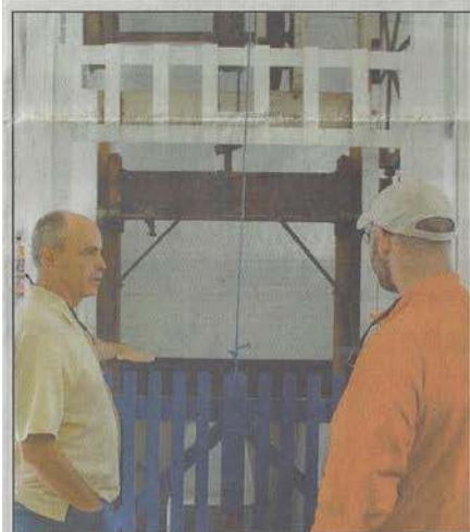
ANDY RODGERS (left) tells a visitor, Joshua Golub of Richmond, about the old-fashioned wooden elevator in the former cement block factory, now Renegade Art Glass, that once carried bags of cement from the railroad level to the second floor. (Kit Huffman photo)
